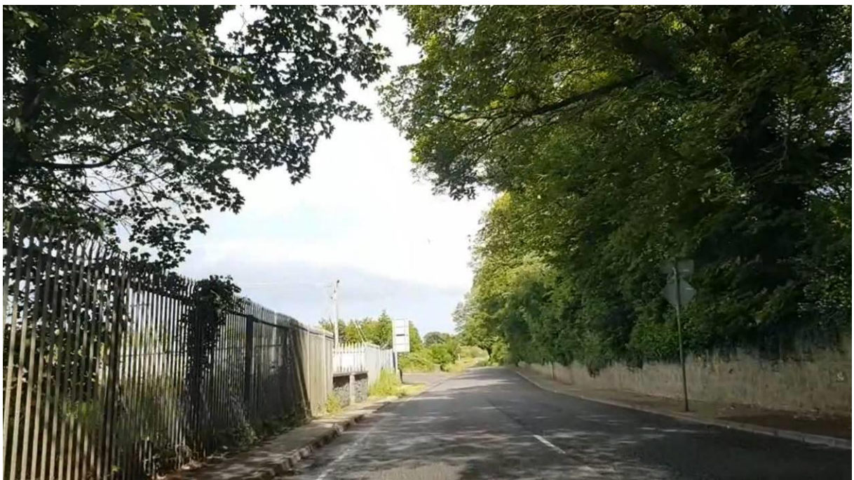
Figure 14: Dense vegetation/mature trees overhanging carriageway on R150
