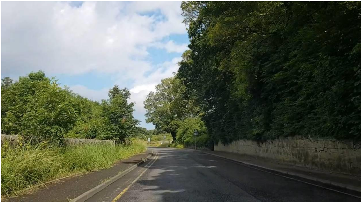
Figure 13: Dense vegetation/mature trees overhanging carriageway on R150
